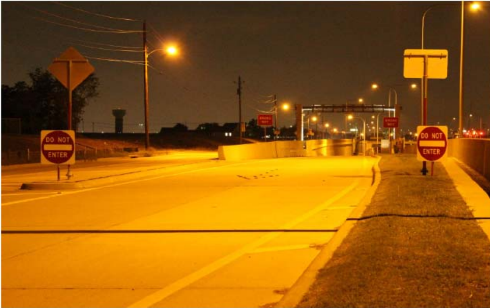
Figure 3. Example of NTTA DO NOT ENTER Lowered Signs. North Texas Tollway Authority (NTTA)
